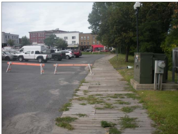
Photo #2-3 (facing north): View of wooden boardwalk with DSMP in the foreground and Bridge Street in the background.
