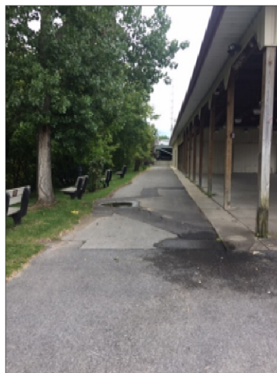
Photo #2-4 (facing south): View of paved portion of the Riverwalk with the PFCM building.
