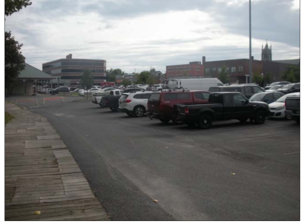
Photo #1-6 (facing southwest): View of the DSMPL with the current Riverwalk in the foreground and the PFCM building, Gateway Complex, Westelcom Suites building, and Clinton County's Department of Social Services building in the background.
