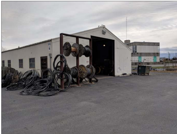
Photo #8-1 (facing east): View of Building 4 at 26 Green Street, with the WRRF in the background.
