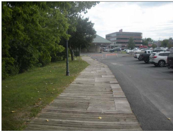
Photo #2-1 (facing south): View of existing Riverwalk, wooden boardwalk.
