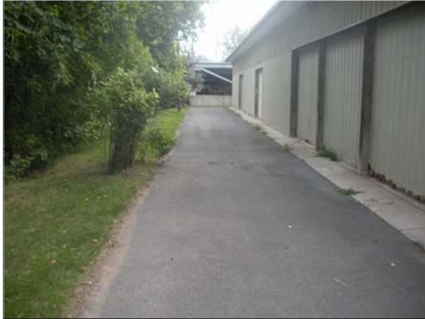
Photo #2-5 (facing south): View of the paved portion of the Riverwalk with the PFCM building and the Gateway Complex's parking garage in the background.
