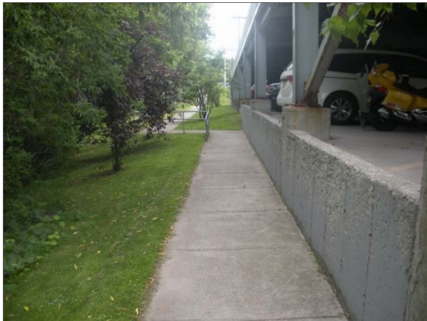
Photo #2-7 (facing south): View of the paved portion of the Riverwalk with the Gateway Complex's parking garage.
