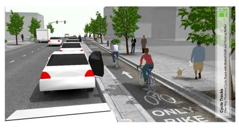
On-street bike lanes with a physical barrier separating the bike lane from motor vehicle traffic. The barrier can include flower planters, concrete curbs, plastic bollards, jersey barriers, and parked cars. Protected bike lanes can be either one-way or two-way.
